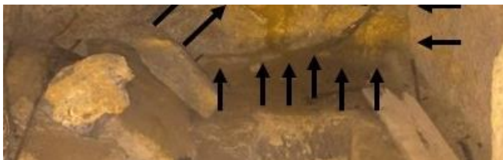
Fig. 4 - Detail of the rear wall–floor junction showing a continuous sub-horizontal interface and localized fine material accumulation. These features are consistent with a potential structural joint. Annotations added by the author for analytical purposes; original image unaltered.
